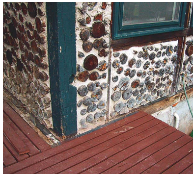
A close look revealed nonexistent insulation, gaping cracks in the cordwood-and-bottle walls and large gable-end holes.
