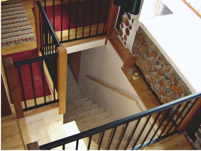
This wide angled stairway to the basement replaced a narrow, open, spiral stairway. The handrail and custom cast-iron railing at the head of the stairs also improved safety.
