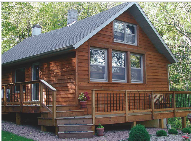
The cedar siding and decks were stained on site to obtain a better finish and to minimize touch-ups.
